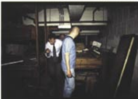
Jack and Doug inspected ALL areas of the Midmer-Losh Organ -- here, they are pictured in one of the sub-stage rooms housing the remains of the combination action equipment.
