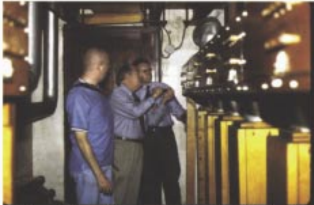
Stephen, Jack, and Doug inspect the method of wiring the windchest of the Pedal Right 64' Diaphone.
