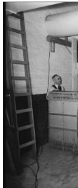
Installing the main console never functioned properly a adjustment. The entire act basement rooms in which
