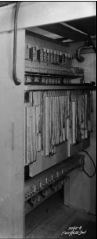
tight Forward chambers. This is organ shop.
