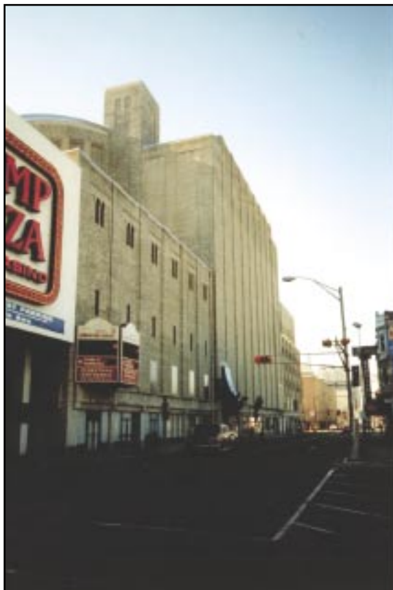
Boardwalk Hall's west end, on Pacific Avenue. The organ shop measures approximately 60ft. x 25ft. and can be seen here behind the single-lancet windows on the left side of the building. Above this, is another room of similar dimensions. This unused room may be a possible location for some of the instrument's blowers — if the suggestion to move them "above sea level" is agreed.
