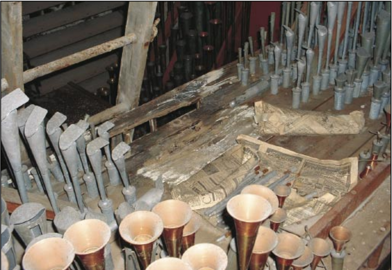
A chest in the Gallery IV organ which, over the years, has sustained considerable water damage. The brass pipes in the bottom of the picture belong to the Saxophone, stop #249.
