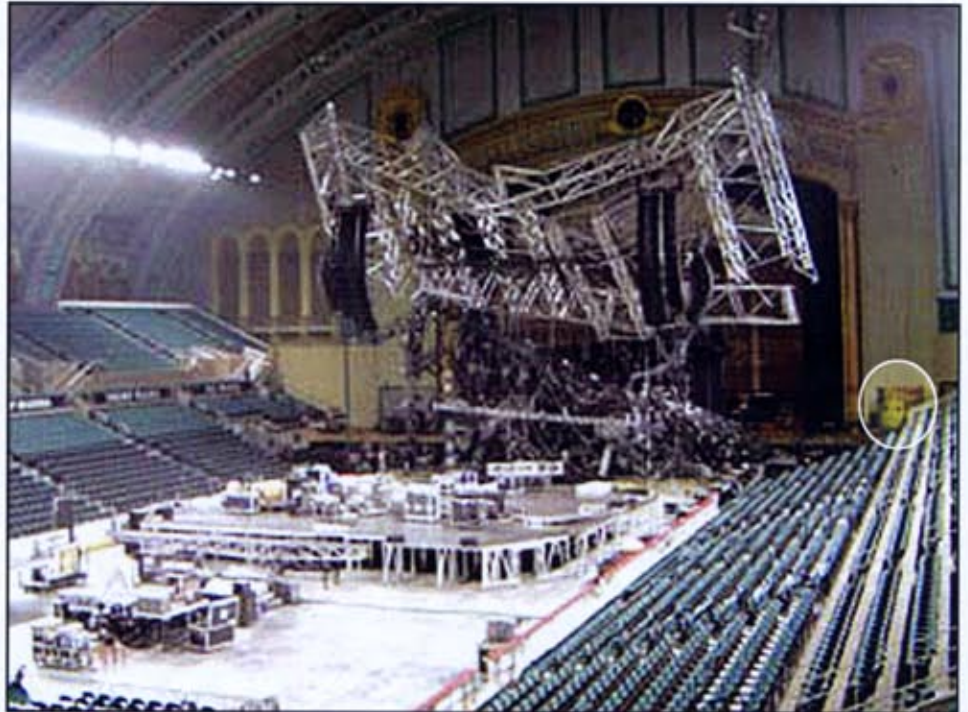
The organ console and kiosk (circled) were out of harm's way.
