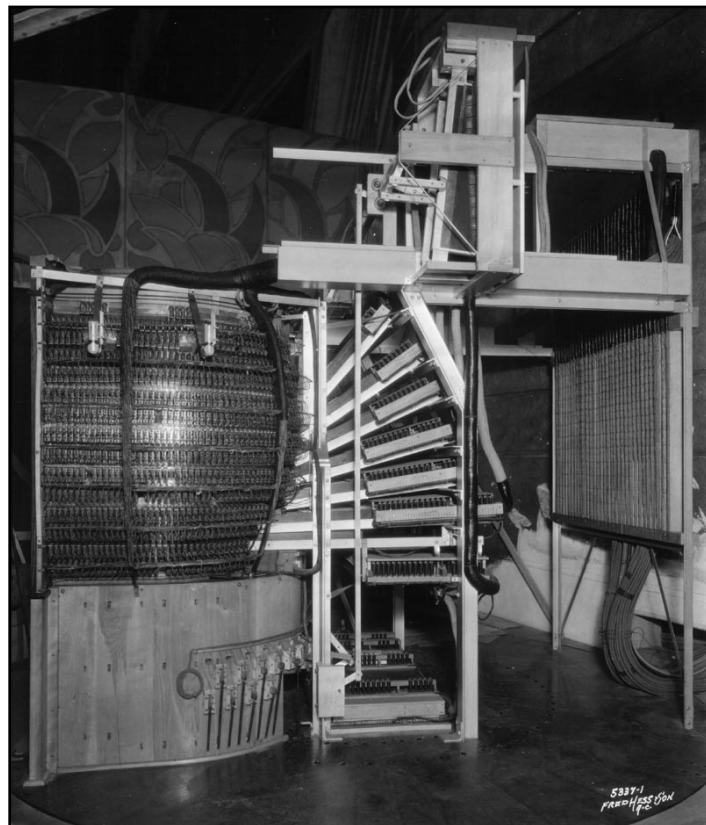
The kiosk encloses all of the equipment seen here. In the center of the picture are the treble ends of the seven manuals at their various angles. Above them are the contactors for the crescendo pedal; these are operated mechanically via the vertical wooden linkage in the center of the photograph. On the left is the back of the console's right jamb and, on the right, is the relay stack. Near the bottom corners of the picture, the edge of the kiosk's revolving dais can be glimpsed. This rotates only a few feet. The frame that supports the manuals, etc., is of aluminum.
