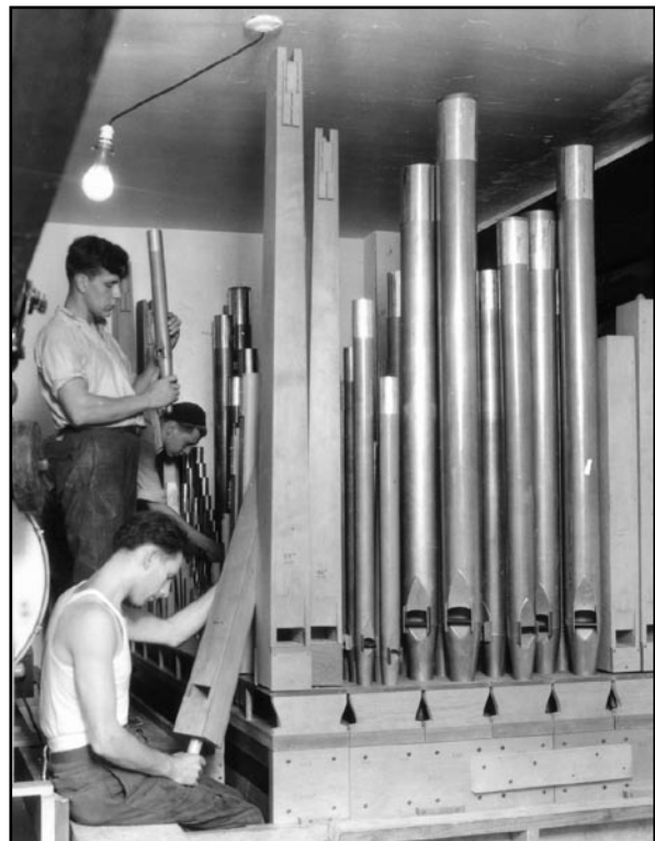
Re. question #39: Here are some of the Swell-Choir's flue ranks being installed, but how many reed ranks does the department have?
