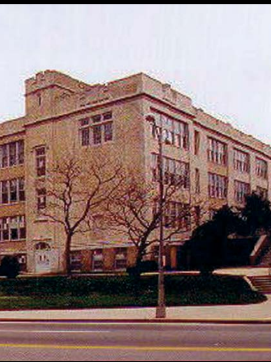
...v been demolished.
