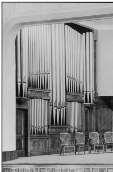
The left case contained the Great and Solo organs, together with some Pedal ranks. Each organ chamber was 26-feet high and contained only pipes — as the blowers and other mechanisms were housed in basement rooms.
