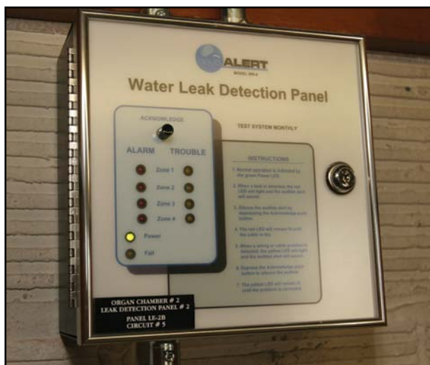
New moisture/water detection panel. Both organs have been fitted with these advanced detection systems.
