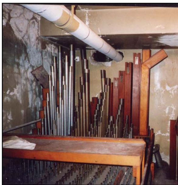
A view of the enclosed Choir organ. Among the stops on this chest are the mixtures (right) and higher-pitched voices. The wooden pipes belong to the extended Melodia rank. Evidence of water damage can be seen on the walls.
