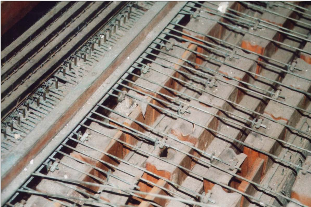
Some of the remains of the remote combination action for the seven-manual console.
