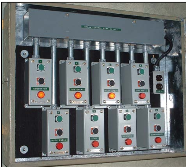
Control panel for the blower motors. From left to right, top to bottom: Generator, Low Great, High Great, Low Swell, High Swell, Echo, Fanfare, Compressor (for the 4 reeds on 100" of wind.)
