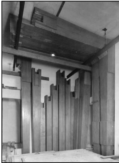
The world’s largest organ pipes. Despite any uncertainty about the 64-foot’s voice, construction and installation of its pipes continued. The longer mitered pipe seen here is CCCCC and to the right of it, nearest the camera, is the CCCCC# (with an extended lower section, so that it is supported by the steel girder). The other flared pipes seen here are also from the 64-foot rank and the straight pipes against the wall are from the 32-foot octave of the Great organ’s Sub Principal.
