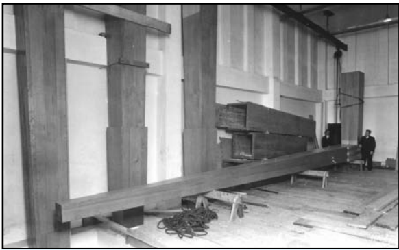
Pipes for the 64-foot stop in various stages of construction. The completed pipe is the 64-foot, and sections of the CCCCC# pipe are stacked horizontally against the wall. To the right of the pipe is one of its builders (name unknown) and on the left is Seibert Losh. Below this platform – which is now occupied by the Solo and Great-Solo departments – are the basses of the Pedal Right stops and some of the Great organ's larger pipes.
