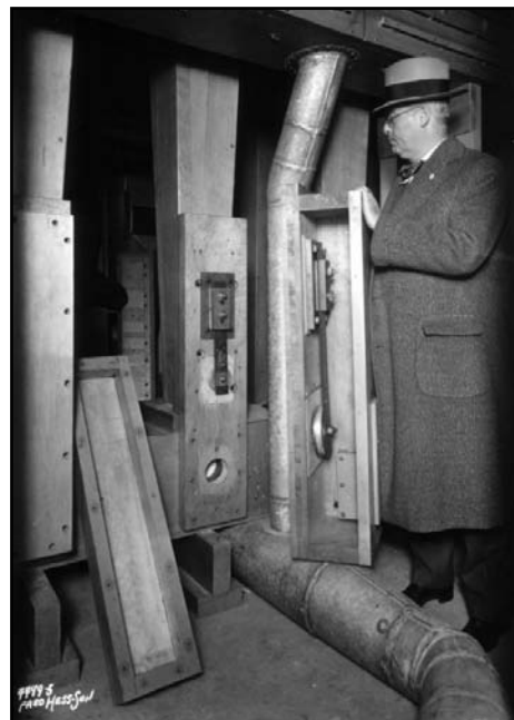
Emerson Richards compares the beaters of large and small diaphone pipes.
