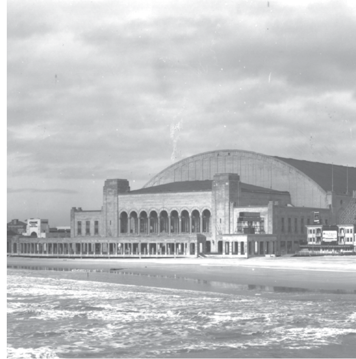
Press photo courtesy of Atlantic City Convention Hall Organ Society Boardwalk Hall, as it appeared in 1929, originally included an open-air loggia that was enclosed when Trump Plaza was built in the 1980s.
